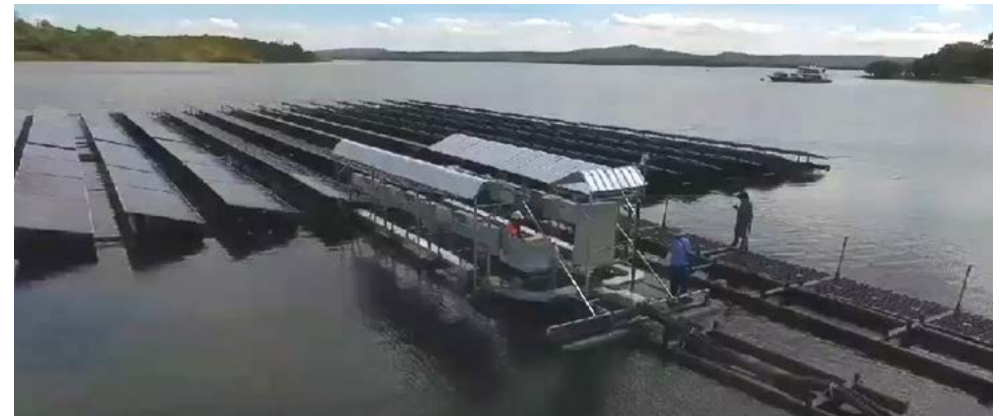
The picture shows the solar power plant project installed on the water at Sirindhorn Dam, size 256 kilowatts
