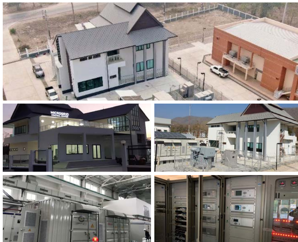
Picture depicts the building that controls the intelligent electrical system, Microgrid development project. Mae Sariang District, Mae Hong Son Province, of the Provincial Electricity Authority
