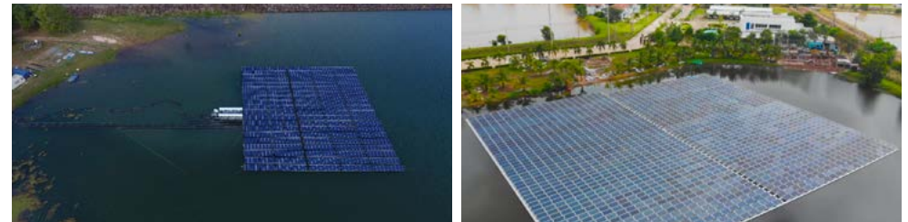
Picture showing the solar power plant project, installed on the water at Prachinburi Glass Industry Co., Ltd. Size 696.80 kW
