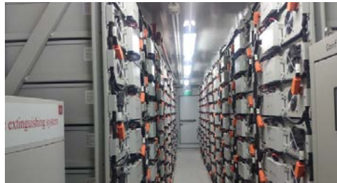
Picture depicts Battery Energy Storage system, size 3 megawatts/2.2 MWh Microgrid development project at Mae Sariang District, Mae Hong Son Province, of the Provincial Electricity Authority.
