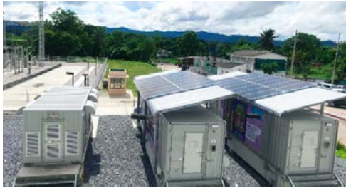
Picture depicts Battery Energy Storage system, size 3 megawatts/2.2 MWh Microgrid development project at Mae Sariang District, Mae Hong Son Province, of the Provincial Electricity Authority.
